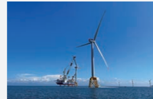
Wind energy generation system (Photo thanks to Green Power Investment Corporation)
