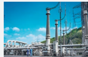
550kV gas insulated switchgear
